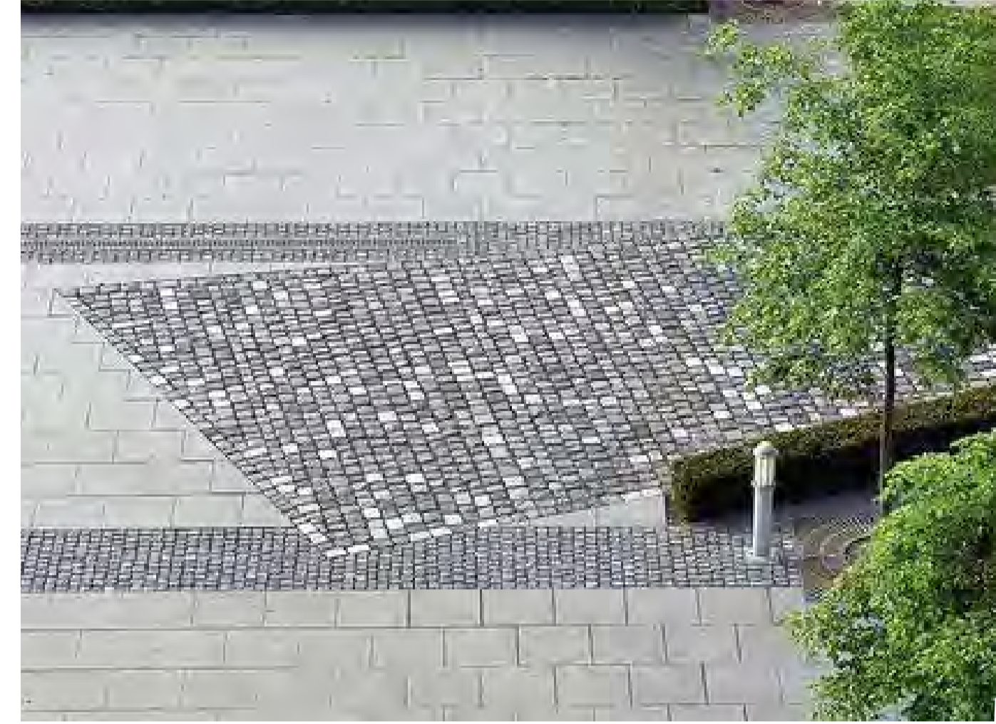
Cobblestone paving to encourage slow and safe riding
